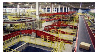
Conveyor-belt sorting system
